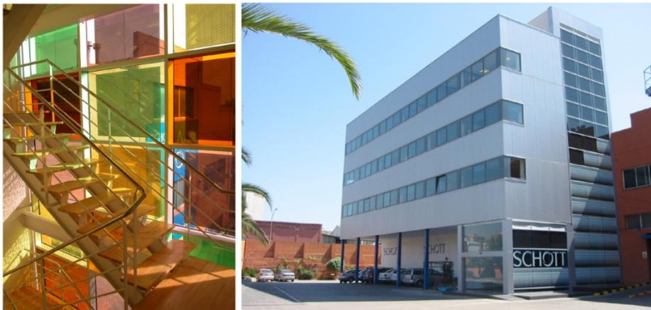
Figure 2.13 Interior view (left) and exterior of finished façade with amorphous silicon PV (Masseck, 2005)
