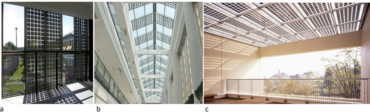
Figure 2.19 BIPV applications in facade (a), skylight (b), and exterior shading like canopies(c)
