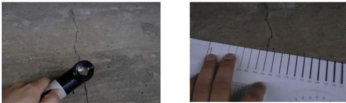
Figure 14: visual inspection site work (Zaki, Murdiansyah & Jusman 2021)
