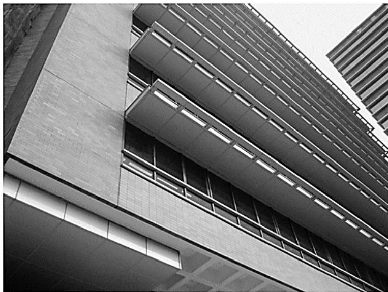
Figure 12: Simple overhang type of external shading (Huang et al. 2011)
