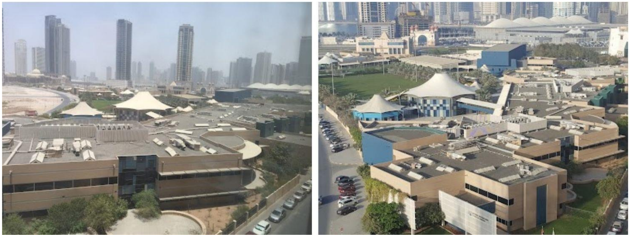
Figure 9: Solar panels at the roof of the VISS school.
