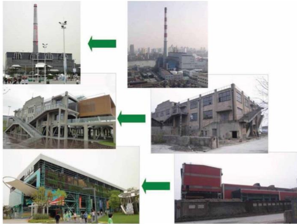
Figure 3.15 Renovation of on-site industrial structures for both Expo and post-Expo uses.
