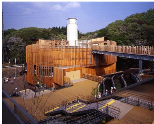
Figure 2.9 the Japanese pavilion using bamboo as a building material (Source: Hikosaka, Y. 2006, p.12)
