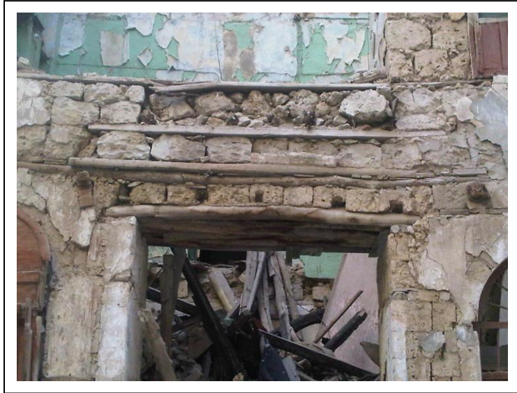
Figure 2-13 Material and Construction Process of the Hejazi house, Author retrieved
