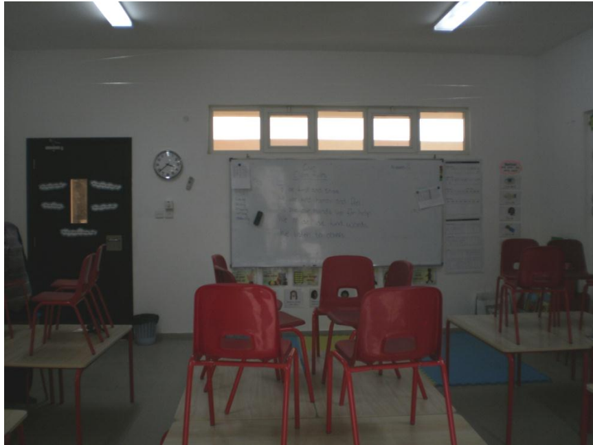
Figure 4-15: Classrooms (A1 and A2) Short Raised Windows (Taken by the author).
