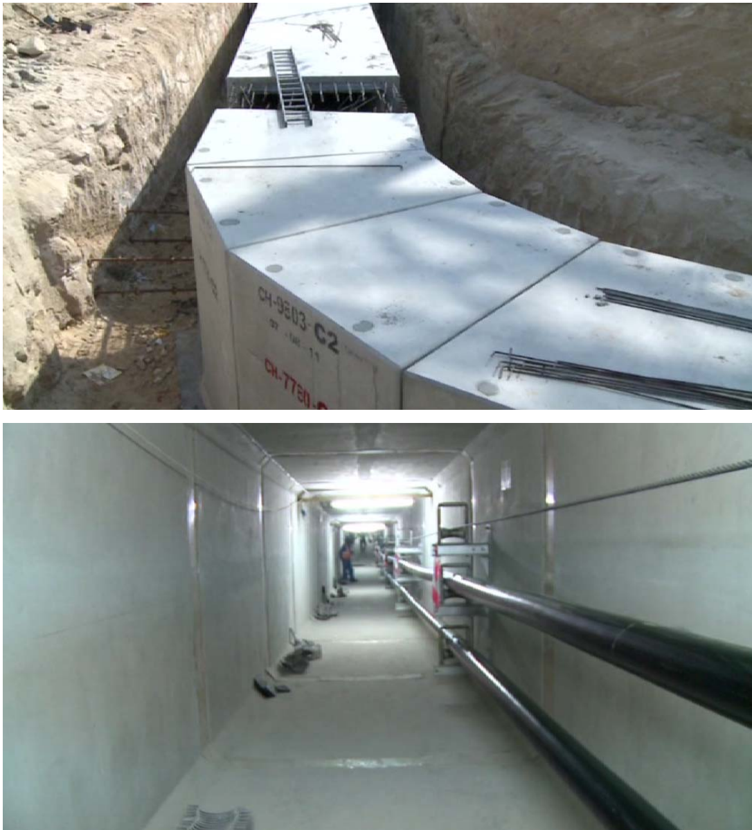
Picture -2: Tunnel (DEWA/Nexan, 2011)
