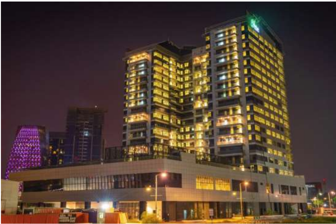
Figure 7; The Y tower Adnec Building.
