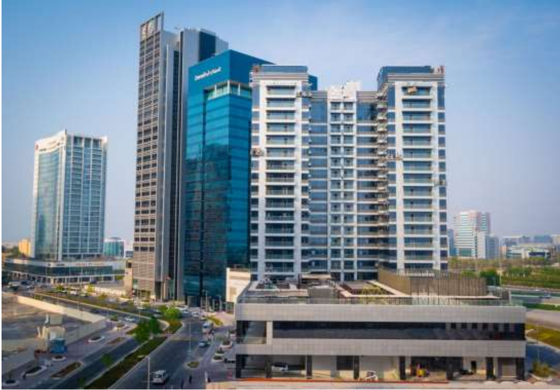
Figure 6; The Y tower Adnec Building.
