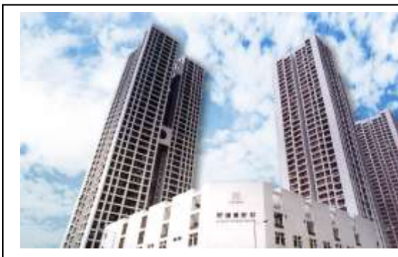
Figure 2.2 Hong Kong high rise public housing. Image source- http://www.housingauthority.gov.hk/en
