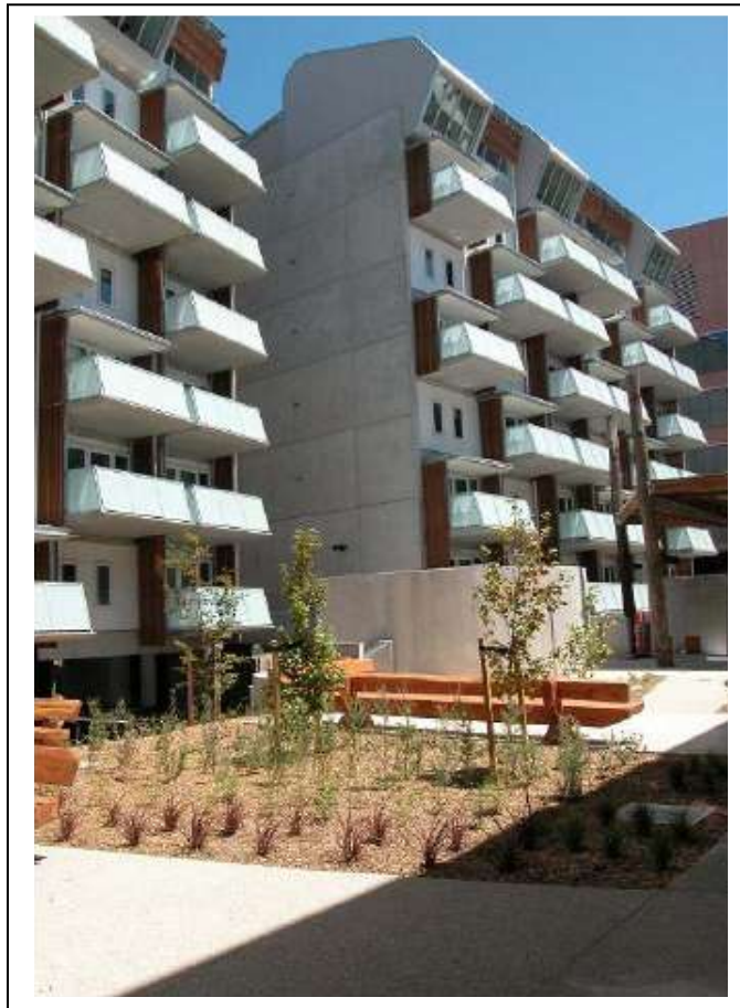
Figure 2.1 Australia’s K2 apartments. Image source- http://www.vic.gov.au/
