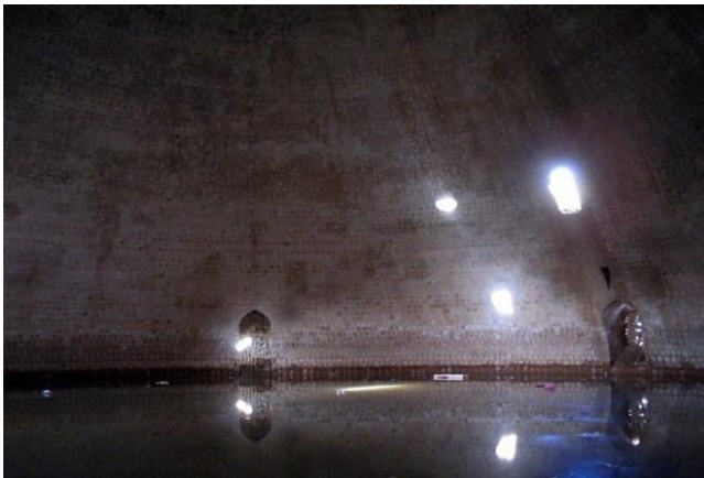
Figure 19: Holes around the cistern (Seeiran, 2011)
