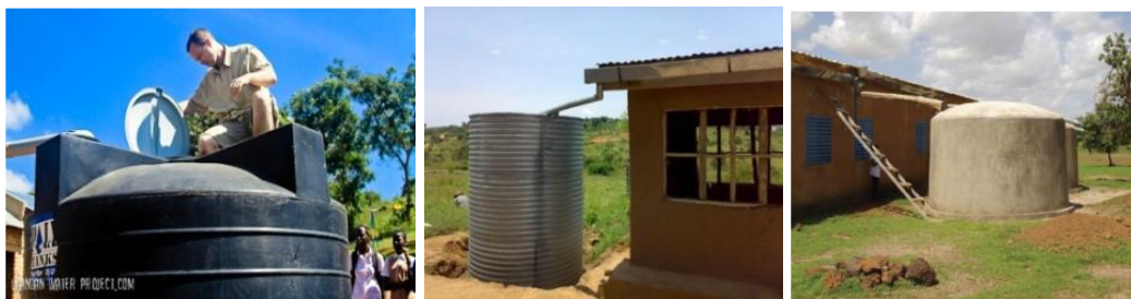
Figure 23: common Rainwater Harvesting and Storage Tanks, Neybare, 2012
