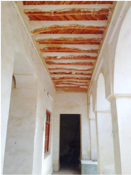
Figure 9: Traditional ceiling design, Evaz, Mirahmadi house, July 2015
