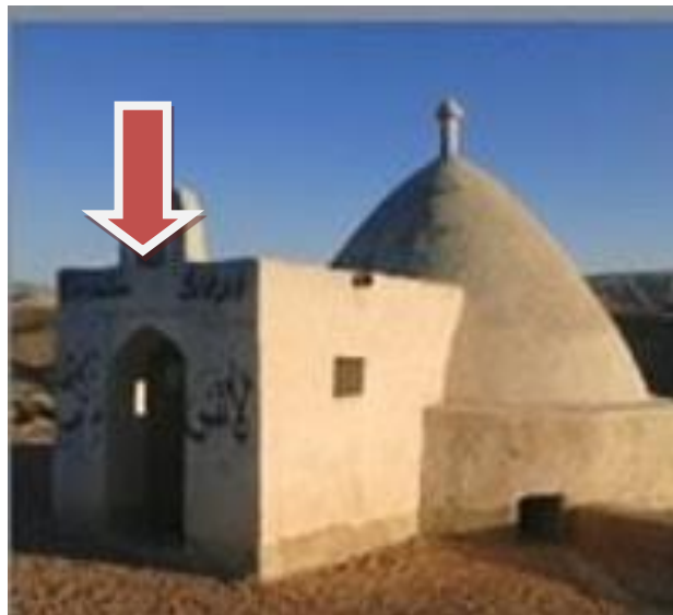
Figure 34-1: The space, which will water filtration, and tank devices locate, by author
