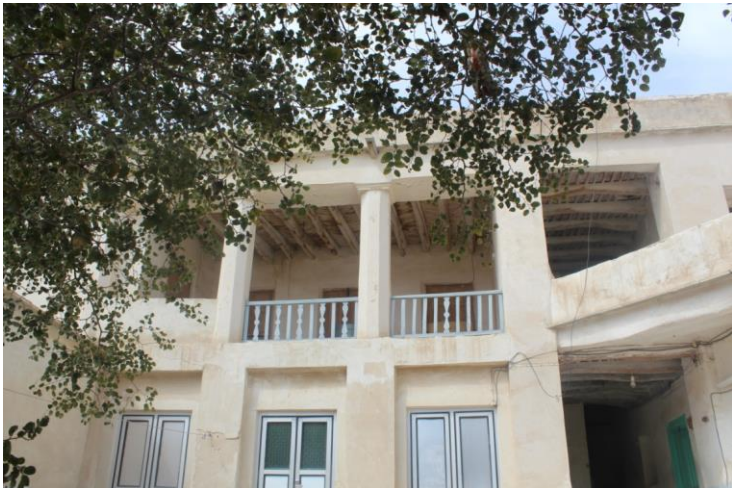
Figure 8: More than 100 years old two story residential building in Evaz; Esmaili Home
