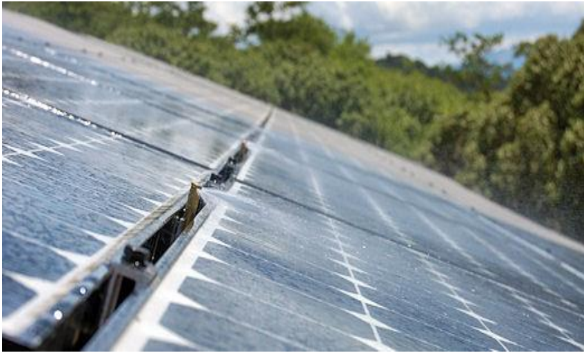
Figure 46: Automatic system of maintenance for solar panel, Solar panel maintenance - the solar company, 2016)
