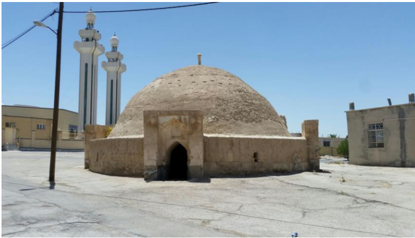
Figure 20: Sheikh's Water cistern, (M.Rahimi, June 2016)
