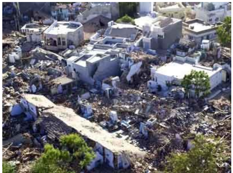
Figure-07: Pictures from Bhuj Earthquake, 2001
