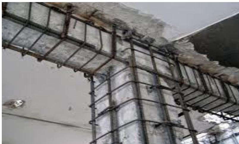
Figure-16: Seismic Retrofitting with Jacketing of Beams
