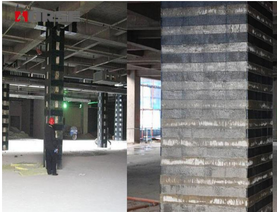
Figure-14: Seismic Retrofitting with Jacketing of Columns using FRP wrapping
