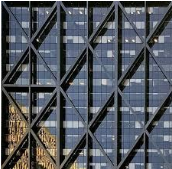
Figure-12: Seismic Retrofitting with Addition of Steel bracings
