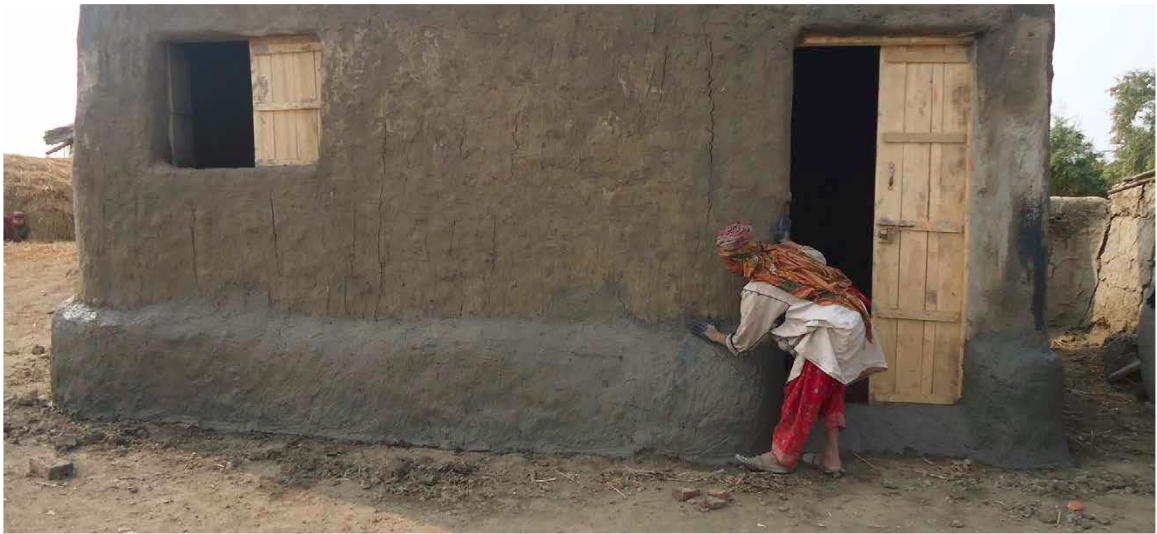
Figure 5: Mud blocks construction (IFRC, UN-HABITAT & UNHCR 2014)
