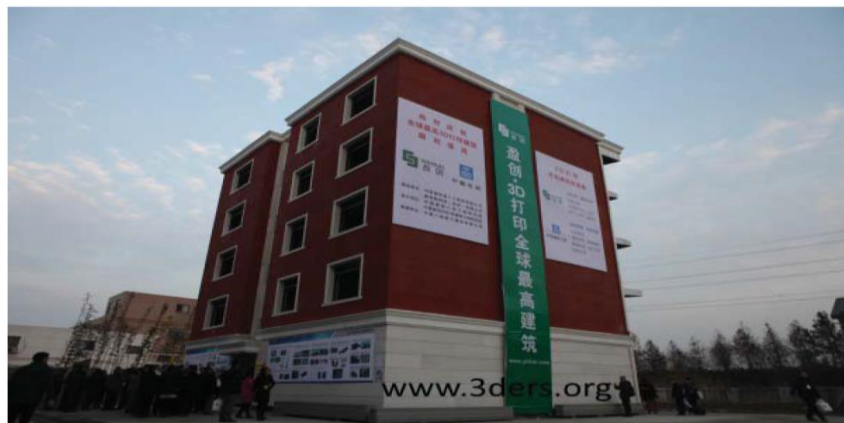
Figure 21 A 3D concrete printed five-story apartment block/ Source: Charron (2015)
