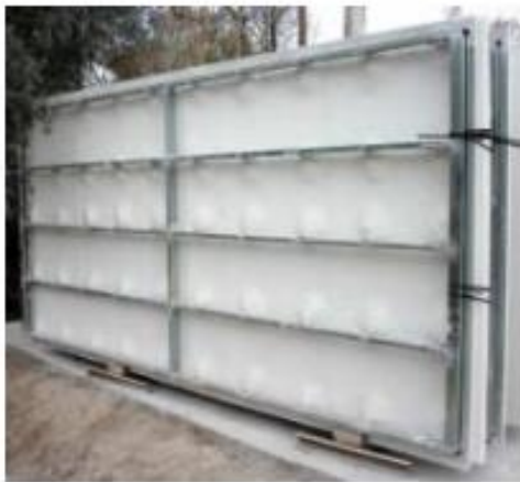
Figure 2 Skin + Stud frame and Ribbed panel / Source (Classen Ungermann and Sharma, 2020)
