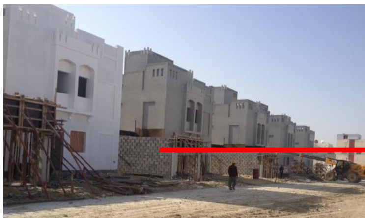
Figure 2.28: Construction method only block work (without insulation) (Source: Author, 2014).
