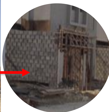
Figure 2.28: Construction method only block work (without insulation) (Source: Author, 2014).
