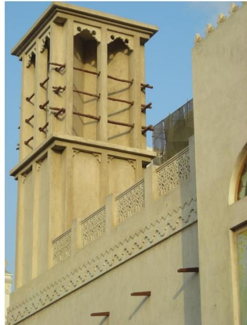
Figure 2.4: Wind catcher in traditional architecture housing design (Author photography)
