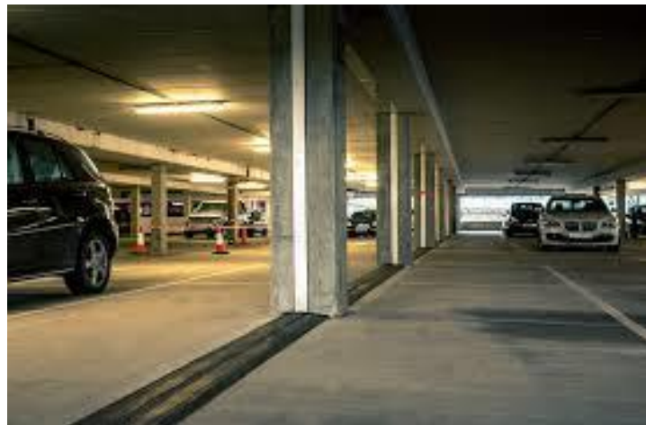
Figure 4.3 Car park expansion joint
