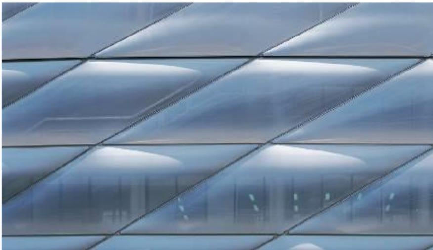
**Figure 2.10. Allianz Arena stadium in Munich with the ETFE envelope (Schittich 2012).**
