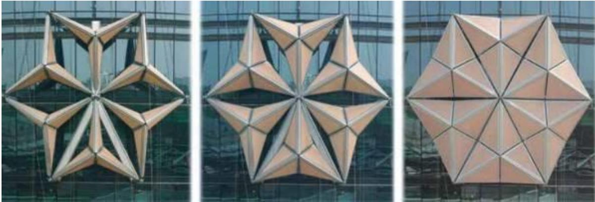
**Figure 2.44. Al Bahr Tower screen different positions (Reid 2013).**
