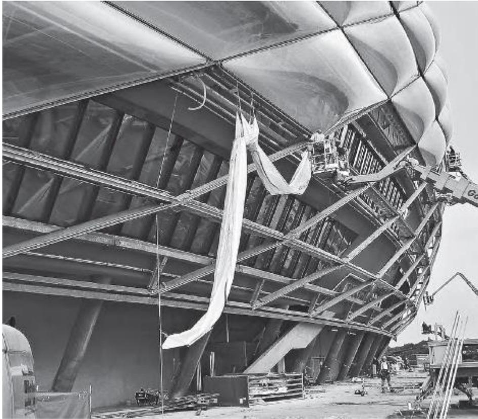
**Figure 2.12. Allianz Arena stadium in Munich with the ETFE envelope (Schittich 2012).**
