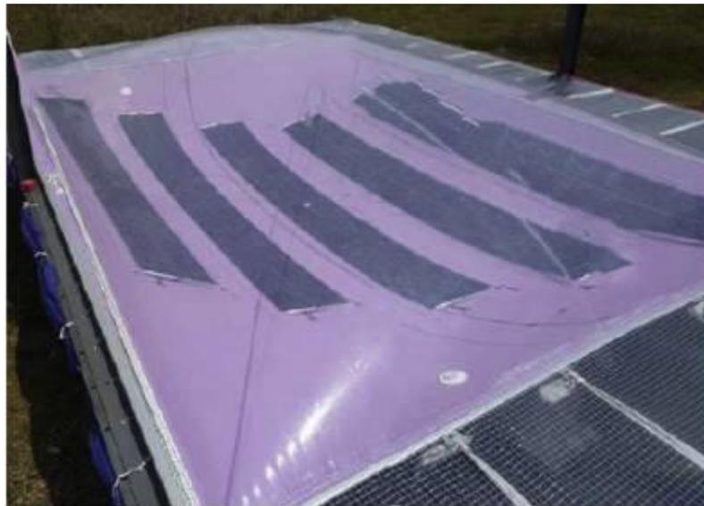
**Figure 2.36. Double layer ETFE with PVs on bottom layer (Hu et al. 2017).**
