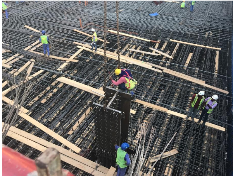
Fig. (1.1) Typical SRC Column Arrangements
