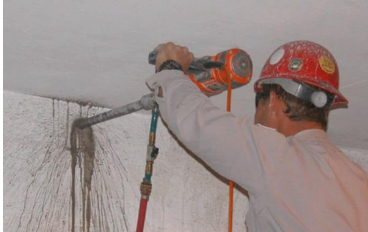
FIGURE 4.14: Coring using Roto-hammer technique (ACI-318, CEU)
