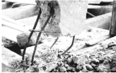
FIGURE 3.6: Structural failure due to lack of confinement (Reinforced Concrete Construction Failures Exposed by earthquakes and other)
