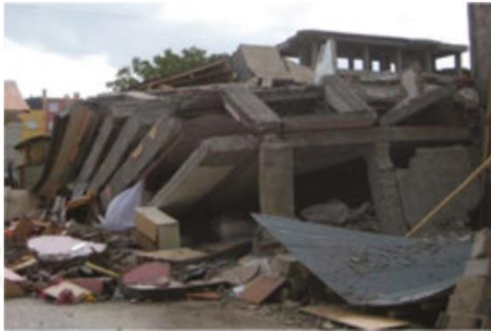
FIGURE 2.12: Strong beam weak column effect causing structural failure (Earthquake & Structural Damages)
