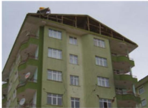
FIGURE 2.13: Gable walls failure on the top of building (Earthquake & Structural Damages)
