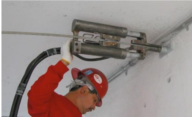
FIGURE 4.16: Stressing of tendons (ACI-318, CEU)
