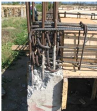
FIGURE 3.11: Improper detailing leading to reinforcement overcrowding (Reinforced Concrete Construction Failures Exposed by earthquakes and other)
