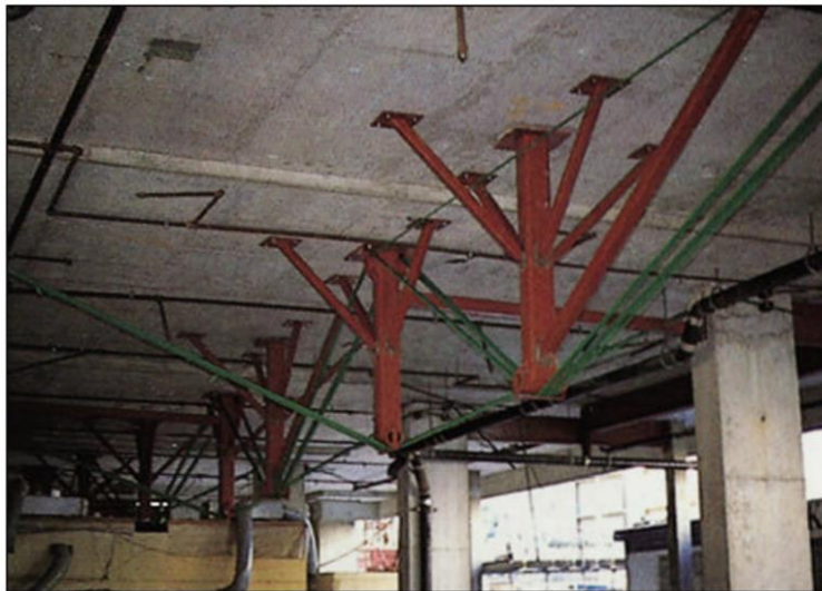
FIGURE 2.23: Representation of saddles and tendons pre fire proofing (Repair & Retrofit using External Post Tensioning)
