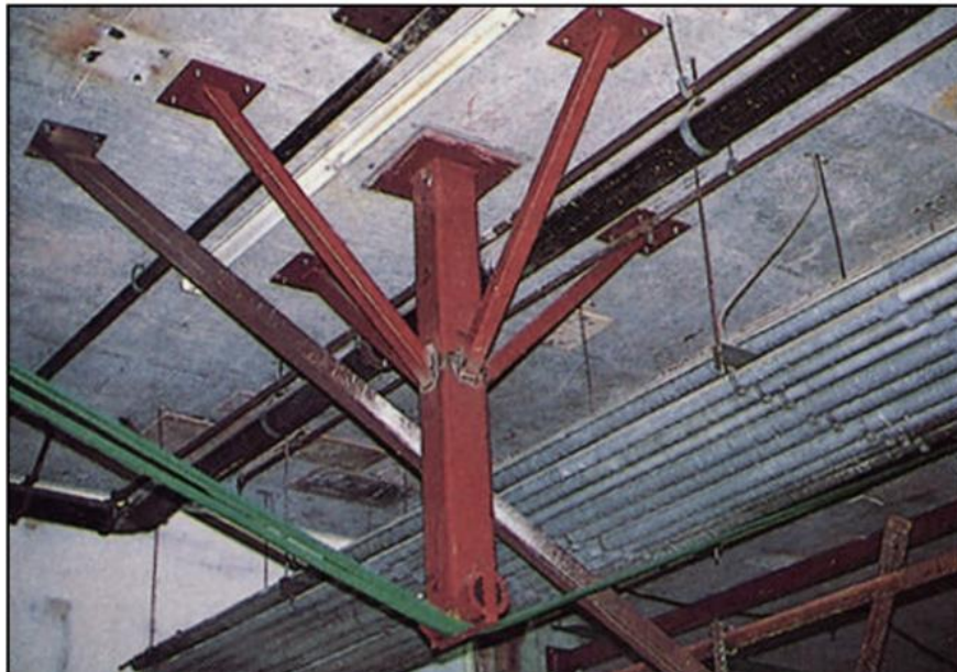
FIGURE 2.19: Arrangements of column saddle after installation of steel tendon (Repair & Retrofit using External Post Tensioning)
