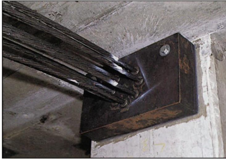
FIGURE 2.22: Typical Anchor plate bearing for the tendon (Repair & Retrofit using External Post Tensioning)
