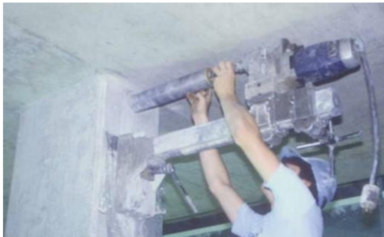
FIGURE 4.15: Coring using special equipment for larger holes (ACI-318, CEU)
