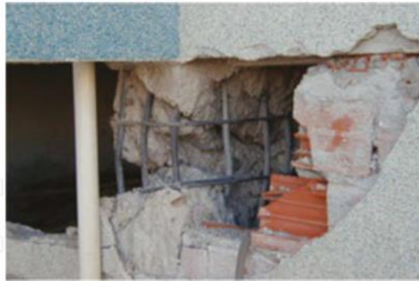
FIGURE 2.10: Representation of damages on short column (Earthquake & Structural Damages)
