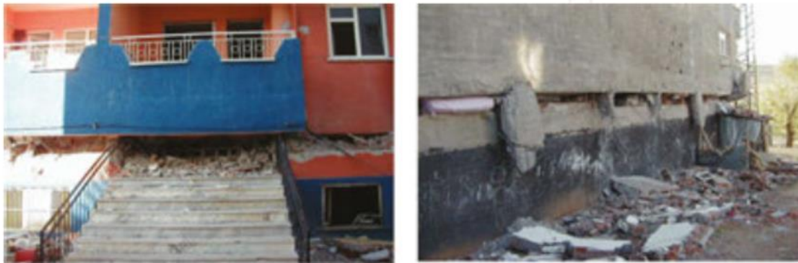
FIGURE 2.8: A representation due to weak story mechanism (Earthquake & Structural Damages)
