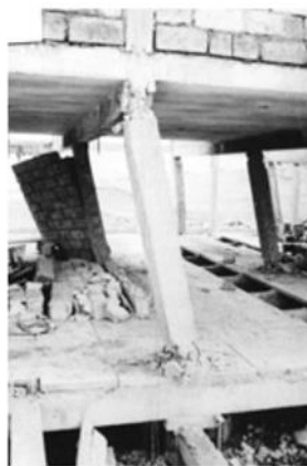
FIGURE 3.5: Structural failure before collapse (Reinforced Concrete Construction Failures Exposed by earthquakes and other)
