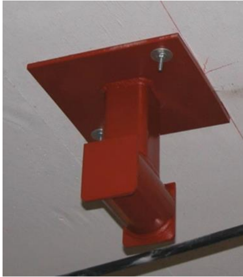
FIGURE 4.8: King post or A-saddle (ACI-318, CEU)
