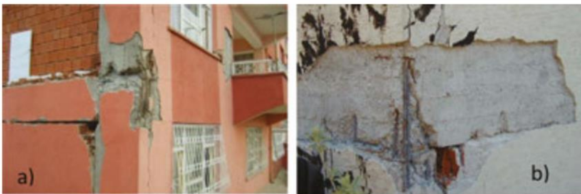
FIGURE 2.8: A representation due to weak story mechanism (Earthquake & Structural Damages)
