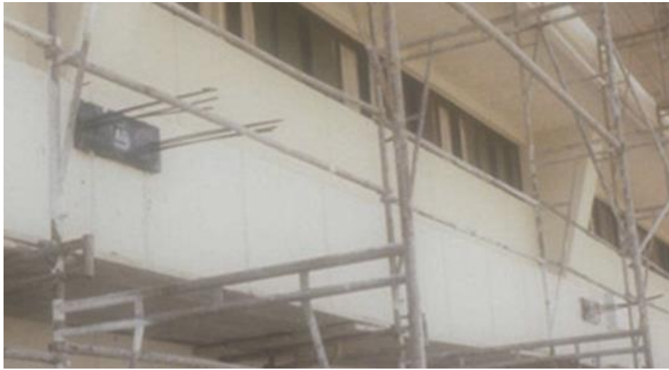
FIGURE 4.19: Anchor bearing plates for tendons (ACI-318, CEU)
