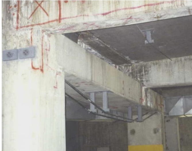
FIGURE 4.12: Strengthening of girders and one-way slabs (ACI-318, CEU)
