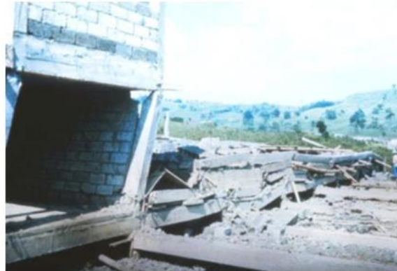
FIGURE 3.16: Modifications by Users without consulting Engineer's absence of shear walls leading to collapse (Reinforced Concrete Construction Failures Exposed by earthquakes and other)
