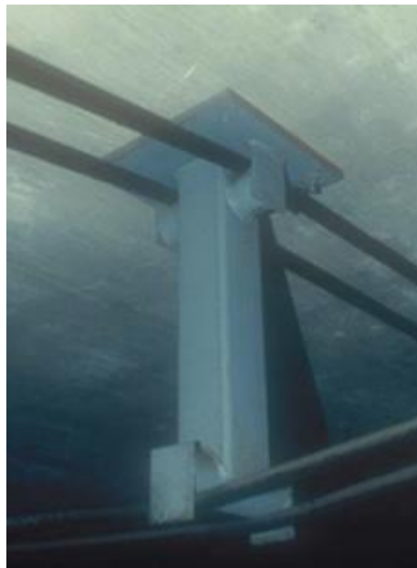
FIGURE 4.9: King post or B-saddle (ACI-318, CEU)
