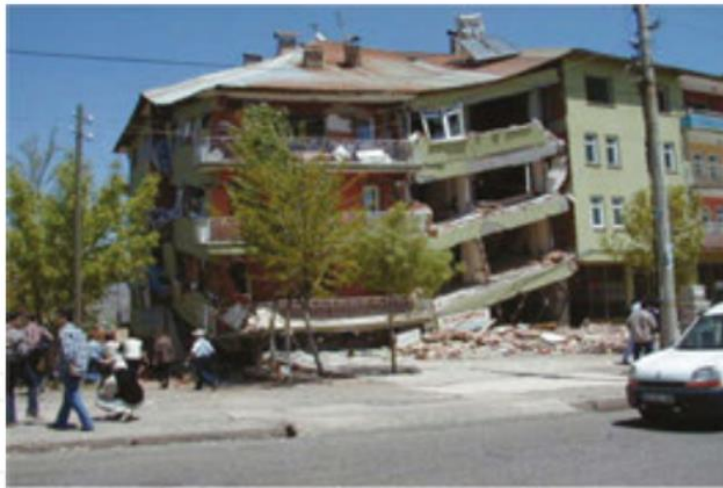
FIGURE 2.11: Adjacent building collapse (Earthquake & Structural Damages)
