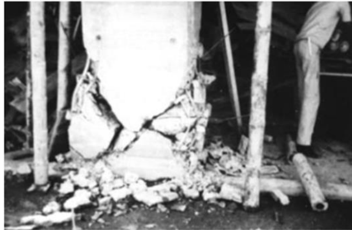
FIGURE 3.19: Improper detailing of column base (Reinforced Concrete Construction Failures Exposed by earthquakes and other)
