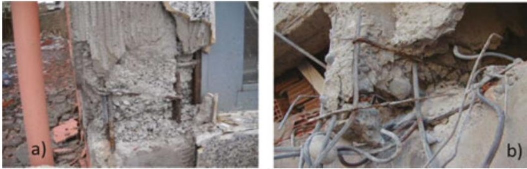
FIGURE 2.14: Poor quality of concrete leading to structural failure (Earthquake & Structural Damages)
