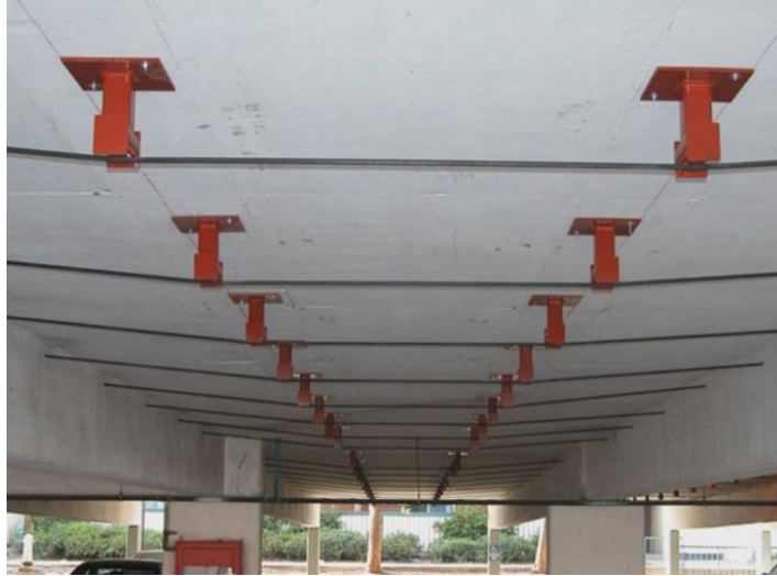
FIGURE 4.10: One way slab strengthening (ACI-318, CEU)
