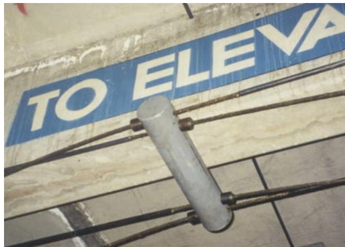
FIGURE 4.17: Method of centre stressing (ACI-318, CEU)
