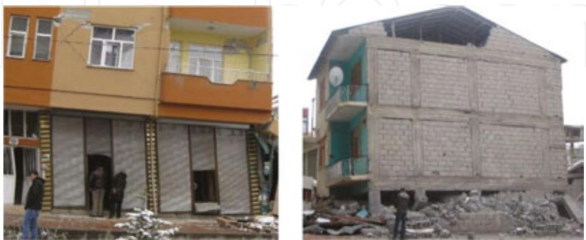
FIGURE 2.7: Soft storey causing unexpected inter storey drift (Earthquake & Structural Damages)
