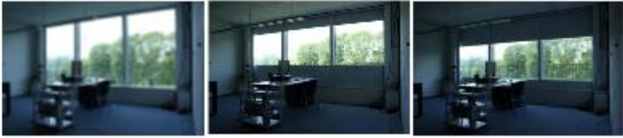
Figure 2.5: shades are fully opened (left). Lower shades are fixed (middle). Upper shades operating only (right) (Bakker et al, 2014).
