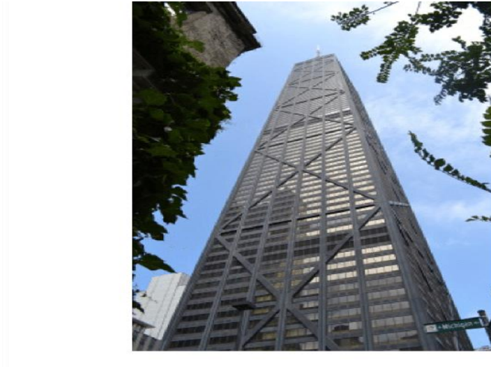
Figure 3: Structural bracing for John Hancock Center building- Sample (Razak et al. 2018)
