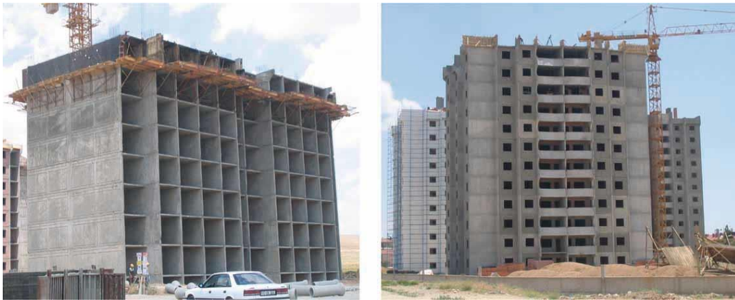
Figure 2: Illustration of shear walls design on site (Balkaya, Yuksel & Derinoz 2010)
