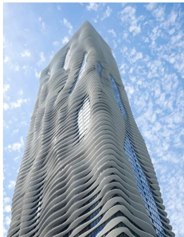
Figure 2.5: static shading devices in Aqua Tower Hedrich Blessing envelope, source: Aqua Tower de Studio Gang | Edificio de Oficinas, 2020.
