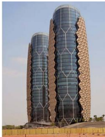
Figure 2.4: kintec shading elements of Al Bahr Towers source: Ltd., Glass, KG and Corporation, 2020.
