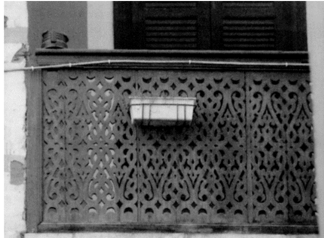
Figure 2.1: Mashrabiya with wooden perforations in one panel source: Ashour, 2018
