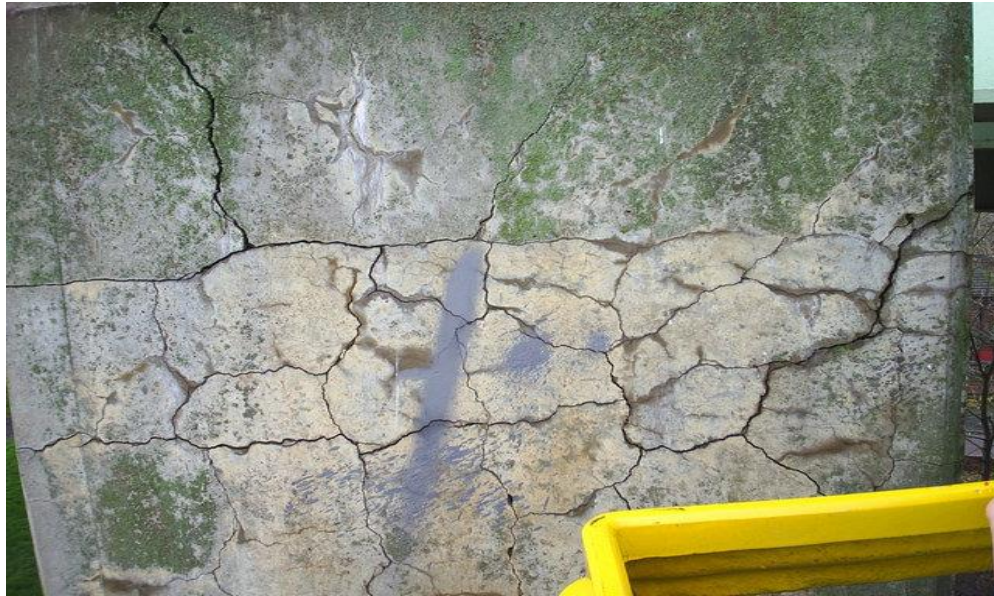
Figure 7 Cracking due to alkali aggregate reaction in Concrete (Brueckner & Lambert 2013)
