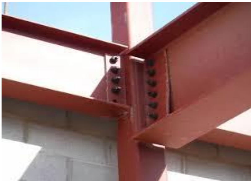
Figure 47: Connection of steel column and beams
