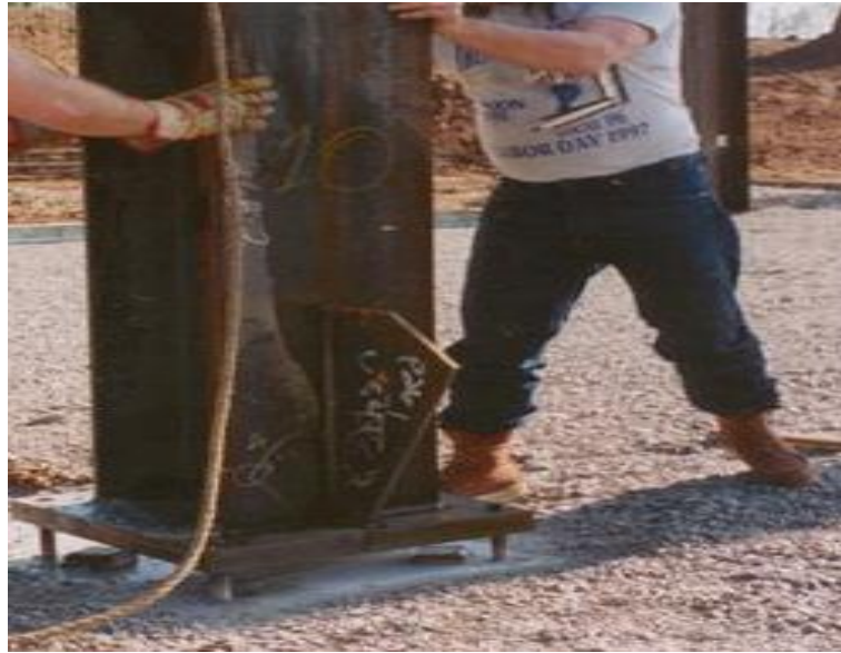
Figure 46: Erection of Steel column
