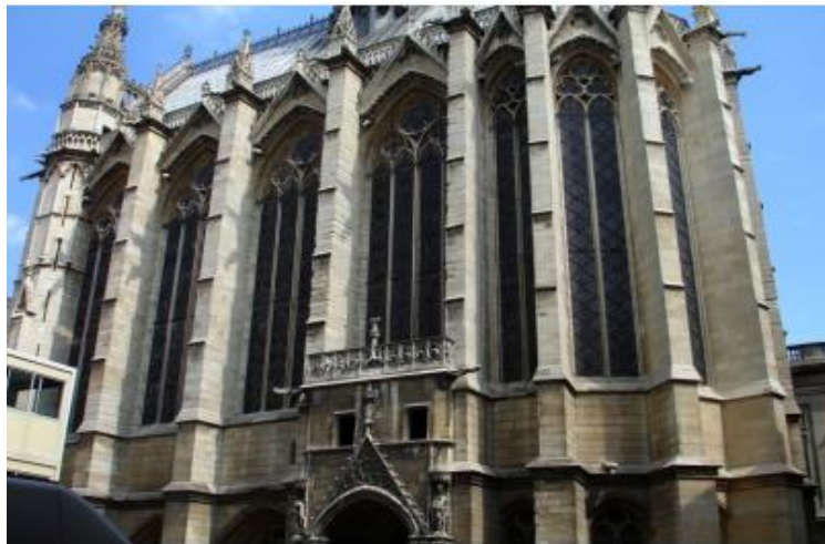
Figure 2.1 La Sainte Chapelle in Paris showing medieval building facade (Cikis 2007).
