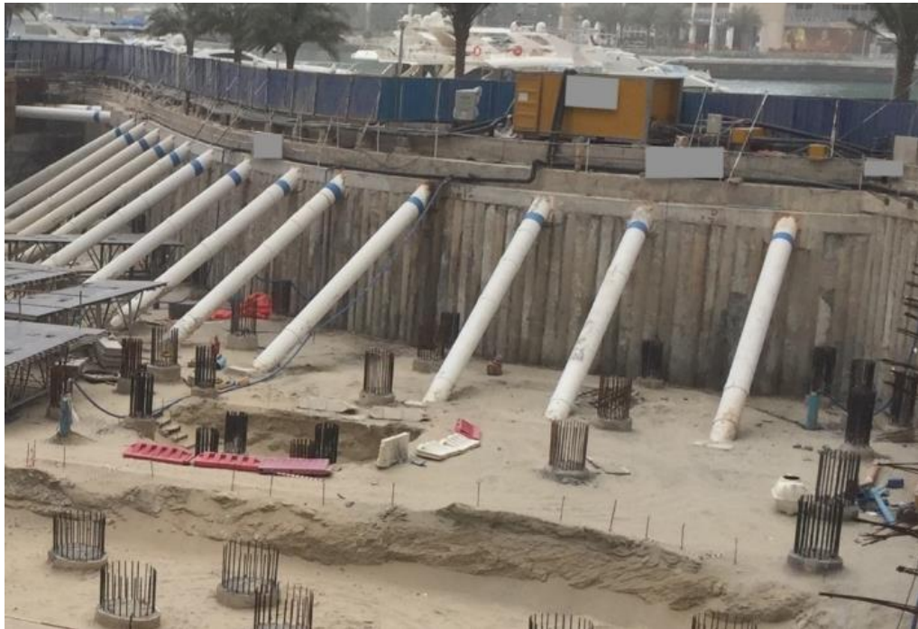
Figure 6 : Inclined struts supporting shoring wall in a construction site(Author)
