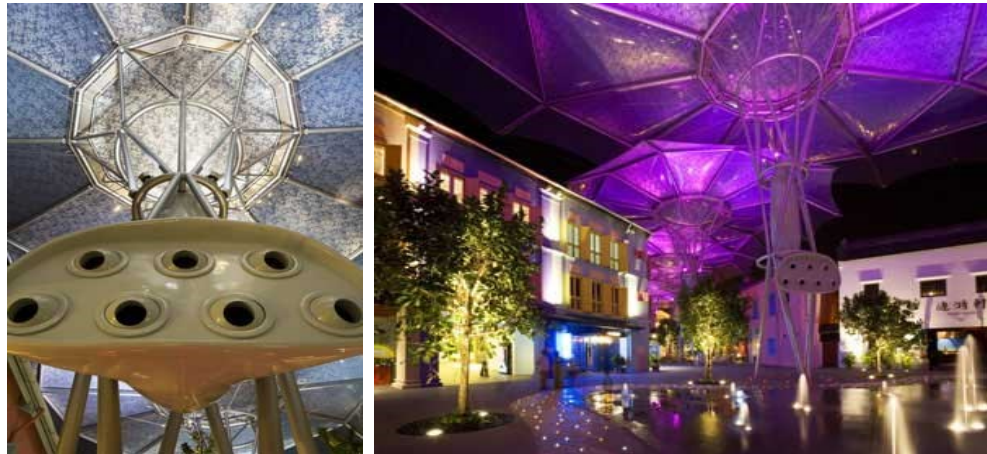
Figure 2.9: The figure showing the mechanical fans within the Canopies. Source: Alsop Architects, 2006)
