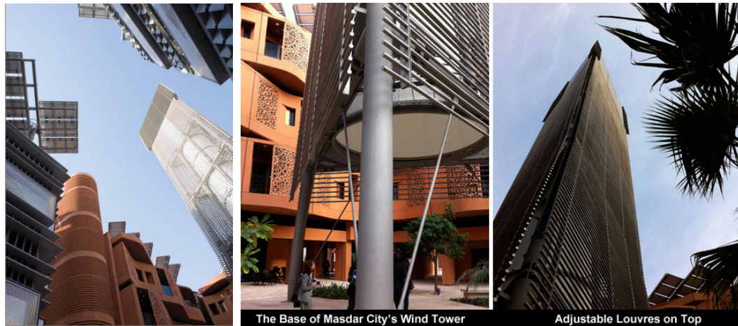
Figure 2.7: Shading devices and wind cooling towers implemented in Masdar City Campus. (Source: images.google.com)
