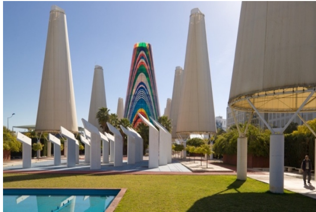
Figure 2.10: The Seville Expo 92, Spain-Avenue of Europe, showing the cooling towers. (Source: images.google.com)
