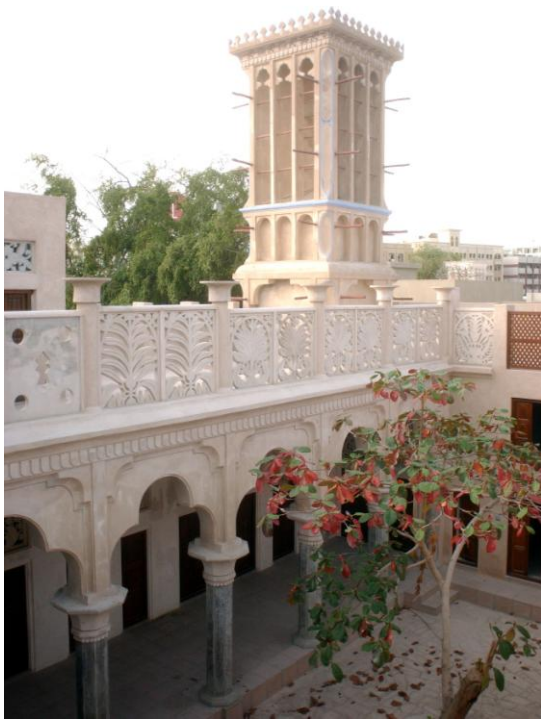
Photo 2.3.5.1 Bastakya wind tower (Dubai architectural heritage society)
