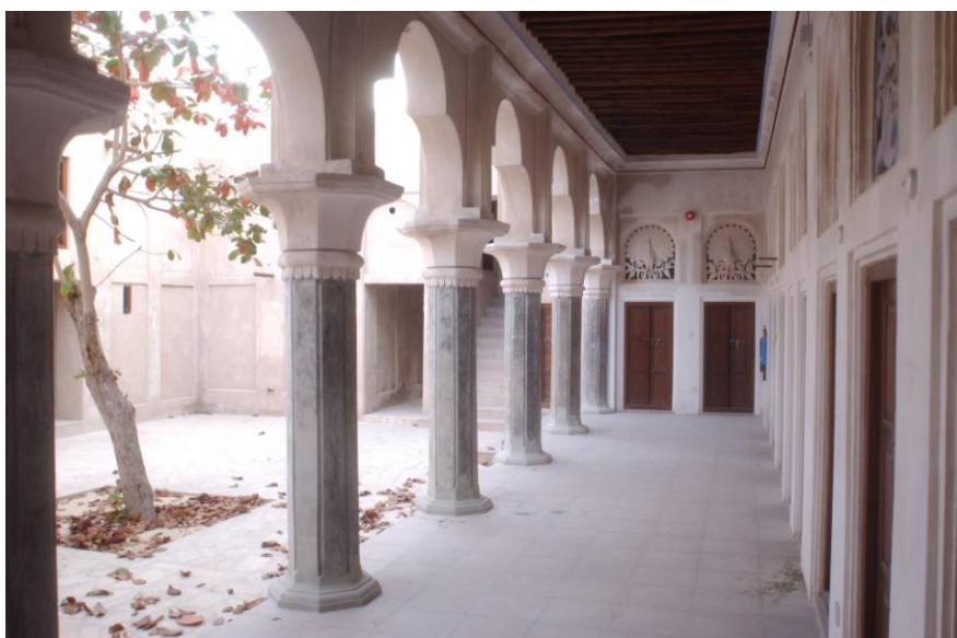
Photo 2.3.7.1 Semi-attached space in the Bastakya courtyard (Dubai architectural heritage society)
