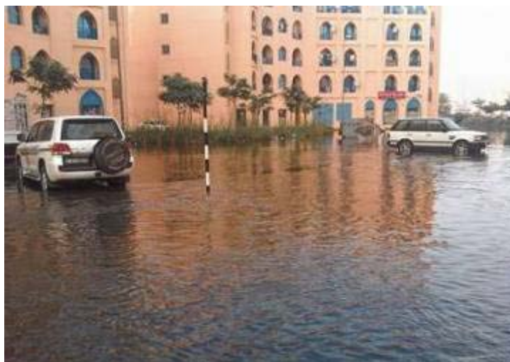
Figure 3: Drainage in Dubai (Gulfnews, January 17, 2011).
