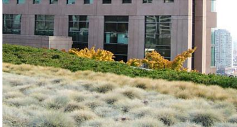
Figure 1.11, Vancouver Public Library: Semi-intensive green roofs are ideal for long-term care facilities, daycare play spaces, employee picnic areas, and urban agriculture, Source ( http://commons.bcit.ca/greenroof/faq.html#6 )
