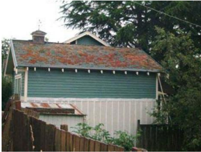
Figure 1.18, The green roof on Tom Balderston's home studio office has a slope of 6.5:12. The slope of this roof posed some challenges for the Northwest Eco Building Guild design team in 2003. Those problems were solved by using circular drainage units, Source ( http://www.pomegranate.org/wp-content/publications/Pomegranate-Center-Greenroof-Manual-2005.pdf )
