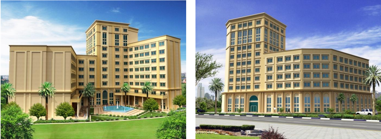
Figure a,b 2.15, Residential Midrise G+M=10, Two different side of the building, Source (Personal Achieve)
