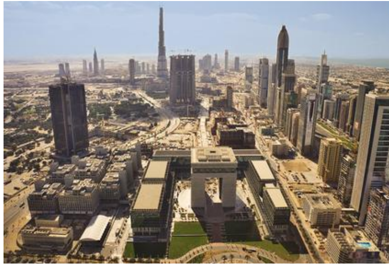
Figure 1.2, Top view of Sheikh Zayed Road Source (Personal Archive)
