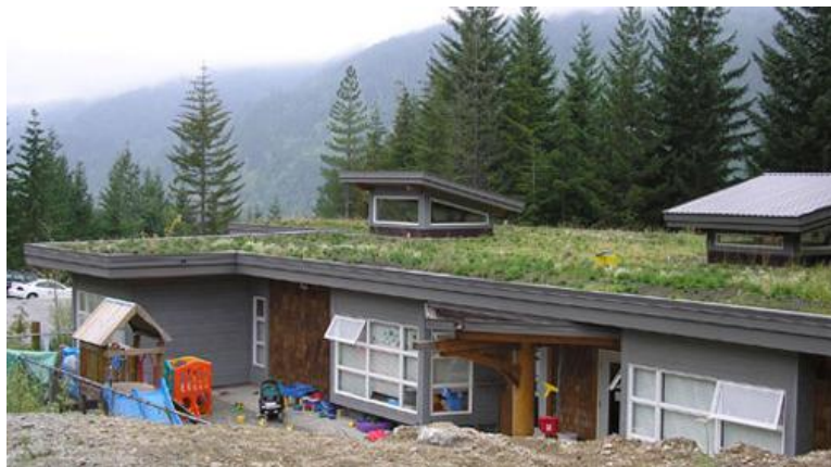
Figure 1.9, Whistler Daycare Centre: Extensive green roofs are ideal for schools, industrial parks, large big-box stores and multi-family housing, Source ( http://commons.bcit.ca/greenroof/faq.html#6 )
