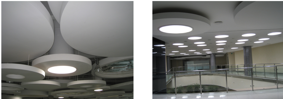
Figure 3.3 Size of Light pipes at Dubai Sales Centre, Dubai, UAE, Personal Archive (2009)
