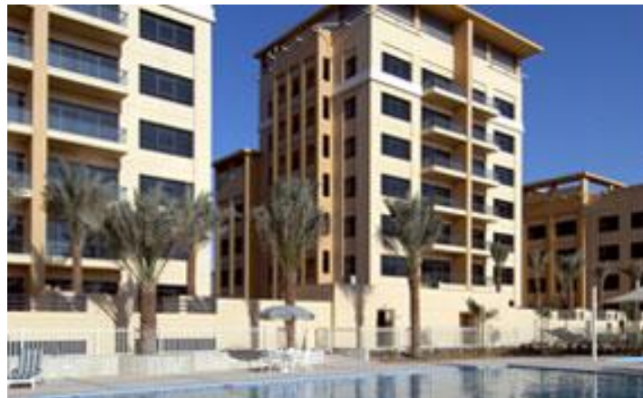
Figure 48. The Greens- Dubai- seven levels (Personal Archive)
