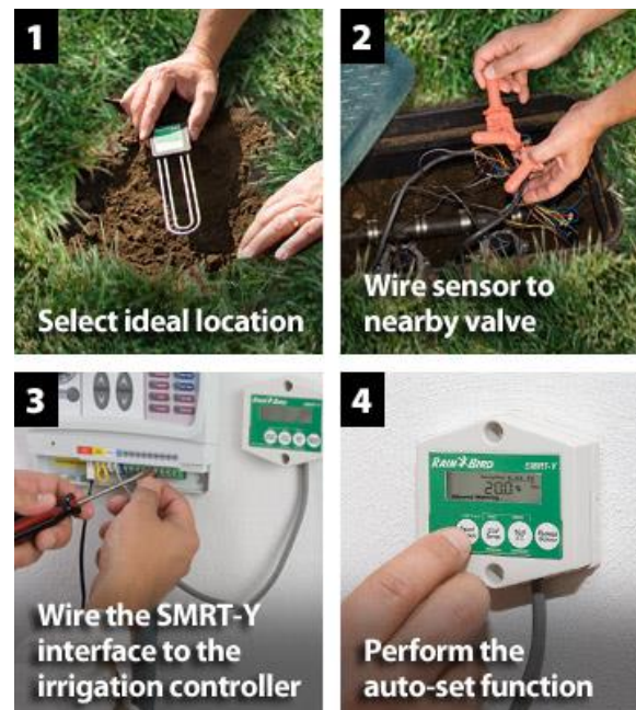
Figure 0.3 The installation of SMRT-Y Soil Moisture Sensor Kit ("Rain Bird SMRT-Y Soil Moisture Sensor Kit" 2017)
