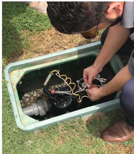
Figure 0.4 Wire Installation on the existing valve (Source: Author).
