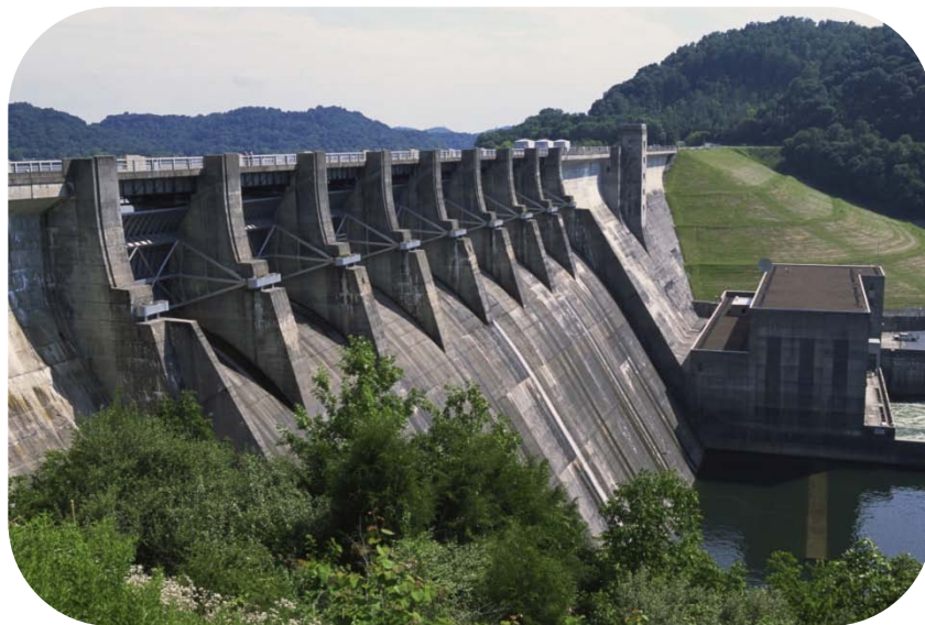
Figure 7 - Electric Generating Dam
