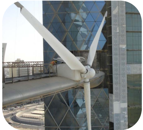
Figure 19 - One of three turbines installed on the BWTC
