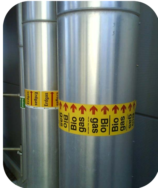
Figure 8 - Biogas processing tubes
