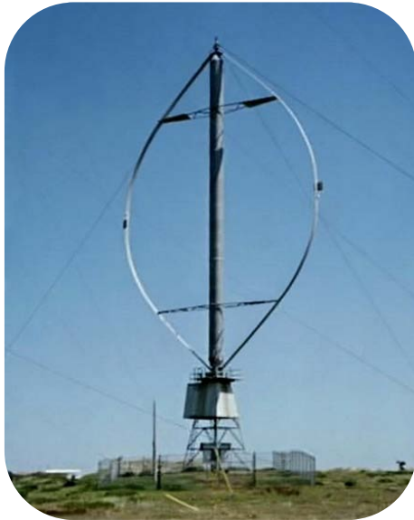
Figure 16 - Darrieus Turbine
