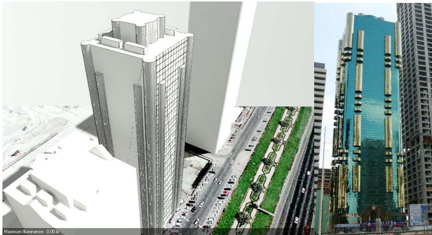
Figure 4.21 (left) Test W.1 daylight illuminance falling on West surface of Al Attar Tower without shading protections (right) Al Attar western facade at SZR (personal archive, August 2009).
