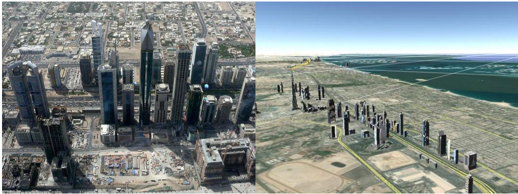
Figure 3.6 (right)Google earth survey show a 78% of SZR offices building s have a square Geometry while 12% were rectangular , 6% circular and 4% triangular. (www.googleearth.com) and (left) Arial view for SZR (www.dubai.ae).
