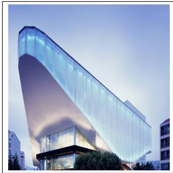
Fig 2.49 Building with ETFE Facade, Image Source- www.makmax.com.au
