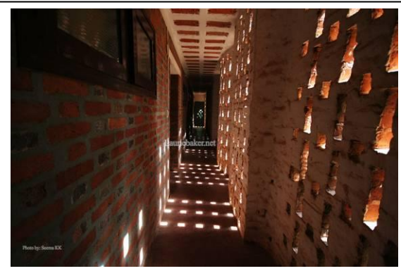
Fig 2.27 Brick Jhalis of Center for Development Studies Image Source- www.lauriebaker.net
