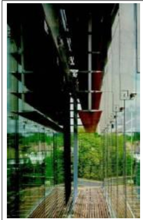
Fig 2.36 Example of Dynamic Shading in Double Skin Facades, Image Source- Bio-climatic facades, Somfy, Living Architecture Conference, Dubai, 19 th Jan 2009, www.somfyarchitecture.com
