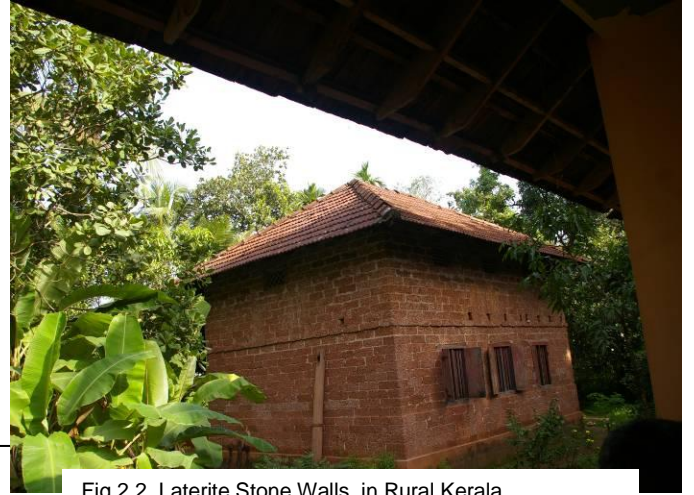
Fig 2.2 Laterite Stone Walls in Rural Kerala, Image Source- Personal Archive- Jidesh Kambil
