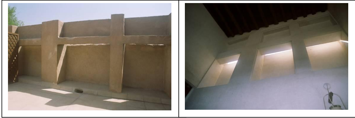
Fig 2.20 Niches in Parapets to direct breeze Image Source- Personal Archive- Jidesh Kambil
