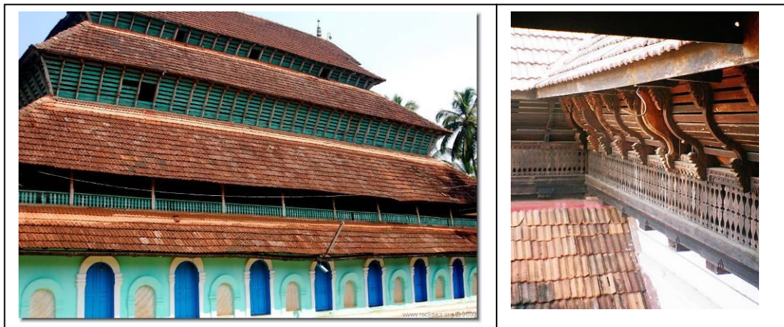
Fig 2.13 and Fig 2.14 Use of Wooden Screens in Facades, Image Source- http://www.rocksea.org/images/kerala ; http://binbrain.com
