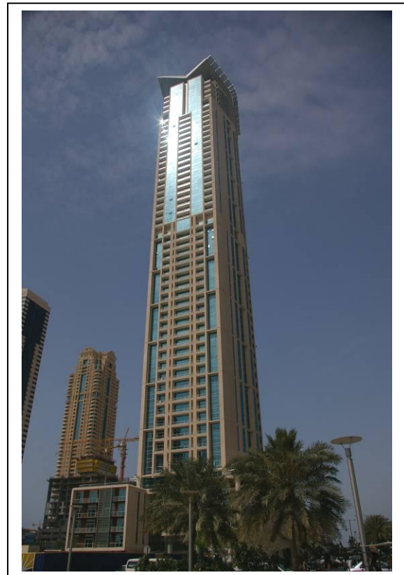
Fig 2.44 Reflected Glare from Glazing on Residential Tower in Dubai Marina, Image Source- Personal Archive- Jidesh Kambil
