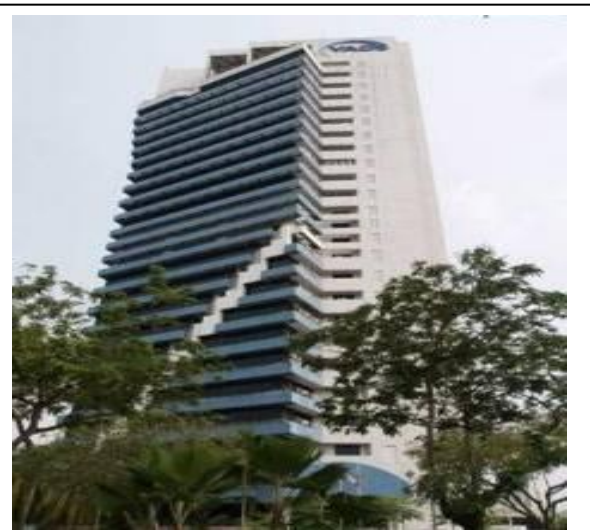
Fig 2.34 IBM Plaza building, Image Source- www.wikipedia.com
