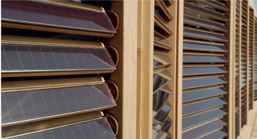
Figure 4-7 Intelligent façade of automatic wood louvers with building integrated photovoltaic panels, TU Darmstadt's 2007 Solar Decathlon House (R. Cole and Z. Brown, 2009).
