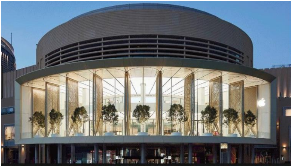
Figure 4-17 Apple Store in Dubai Mall, Dubai ("Apple Dubai Mall with one of the world's largest kinetic art installations| Foster + Partners" 2017).
