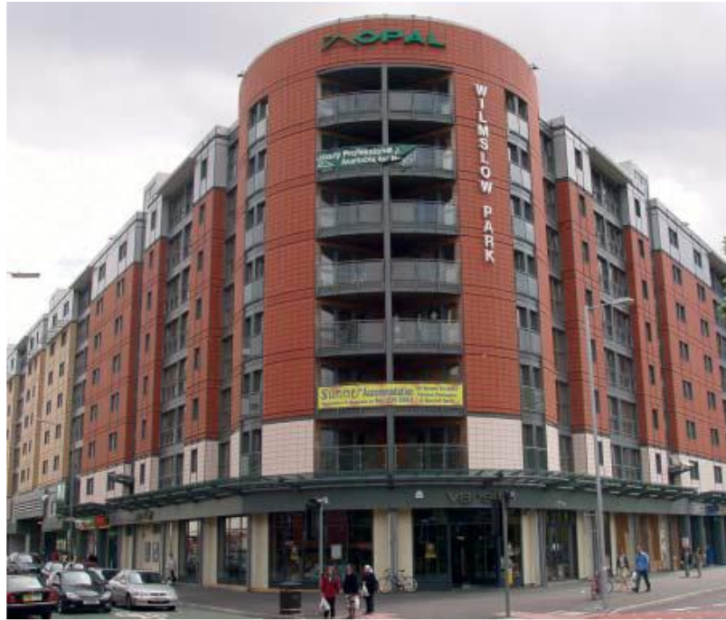
Figure 2.12: Mixed Commercial Residential Development at Wilmslow Road, Manchester, (Lawson et al, 2005)
