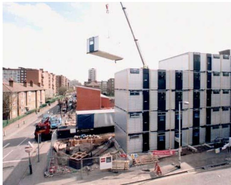
Figure 4.14: Installation of Modular Units at Murray Grove, Hackney (Lawson Et Al 2005)
