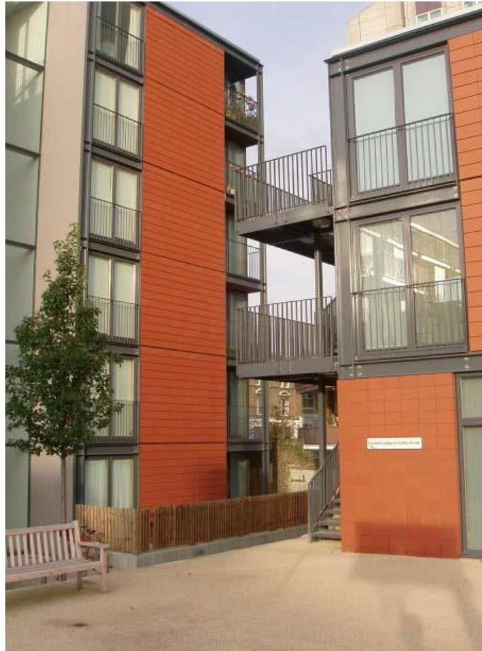
Figure 2.10: Completed Mixed Panel and Modular Project At Lillie Road, Fulham (Lawson et al, 2005)
