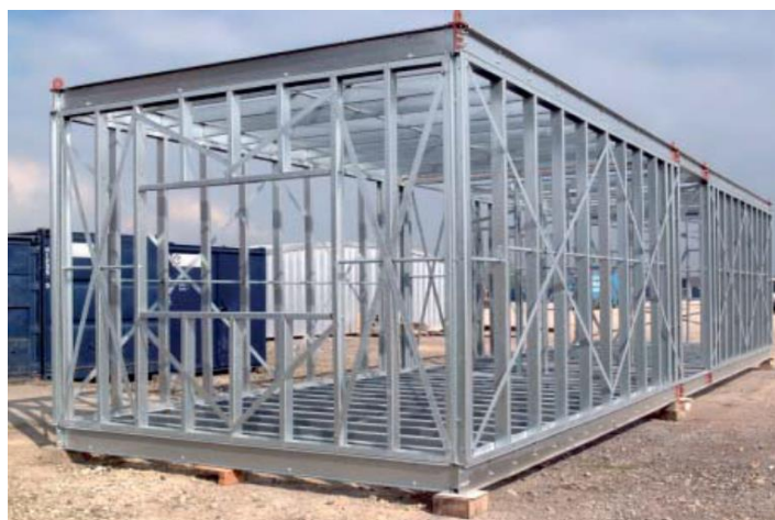
Figure 2.7: Continuously Supported Module in Light Steel Framing (Lawson et al, 2005)
