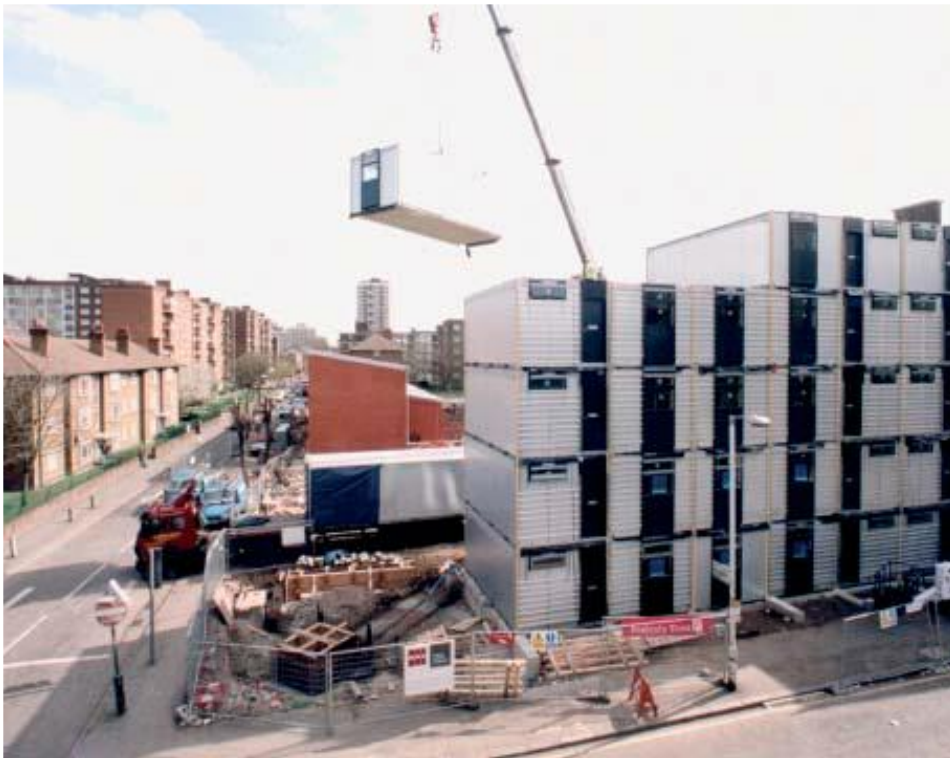
Figure 2.9: Installation of Modular Units at Murray Grove, Hackney (Lawson et al, 2005)
