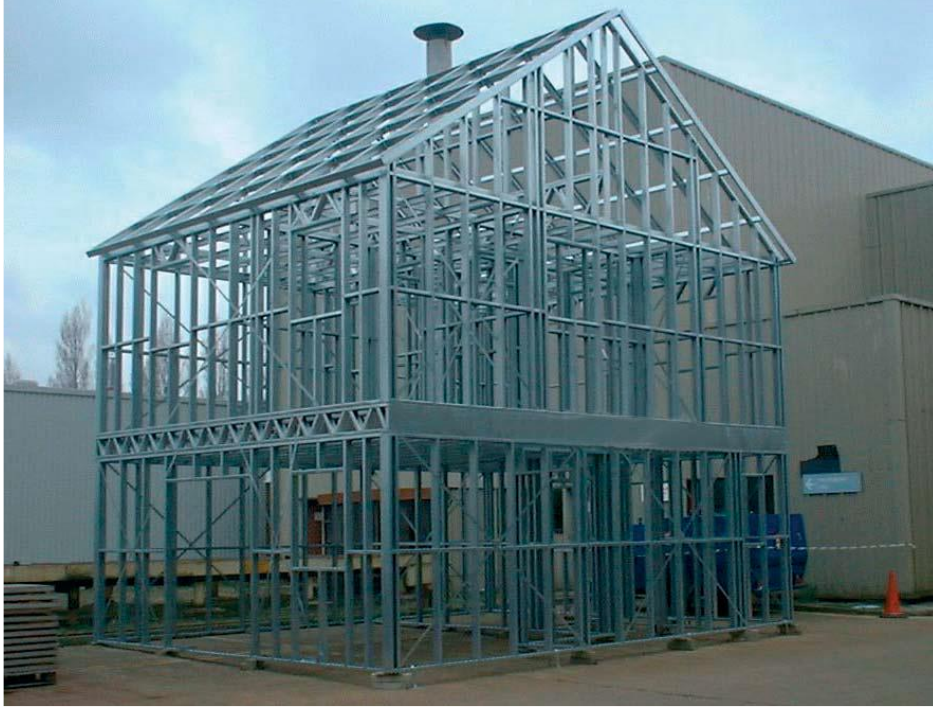
Figure 4.15: Light Steel Framing for Housing (Lawson et al. 2005)
