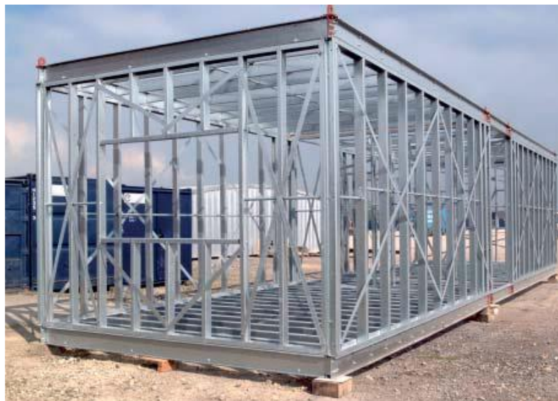
Figure 4.17: Corner Supported Module in Light Steel Framing (Lawson et al. 2005)
