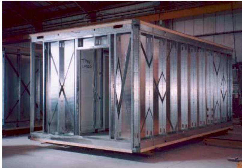
Figure 4.16: 4 Sides Supported Module in Light Steel Framing (Lawson et al. 2005)
