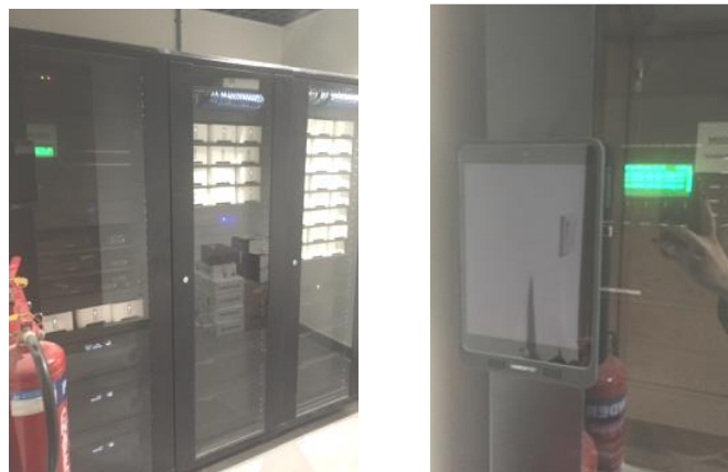
Figure 4.46 Servers' room and Servers control touch screen
