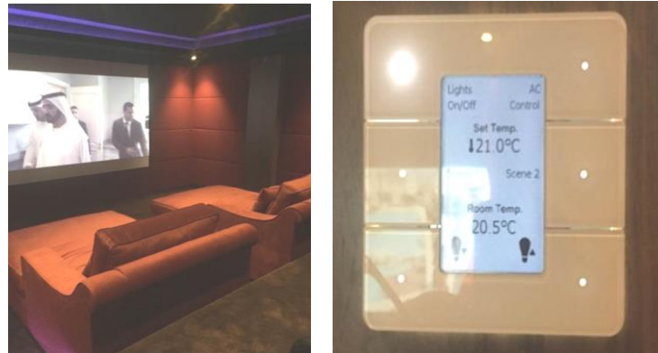
Figure 4.45 Cinema Room control Touch screen
