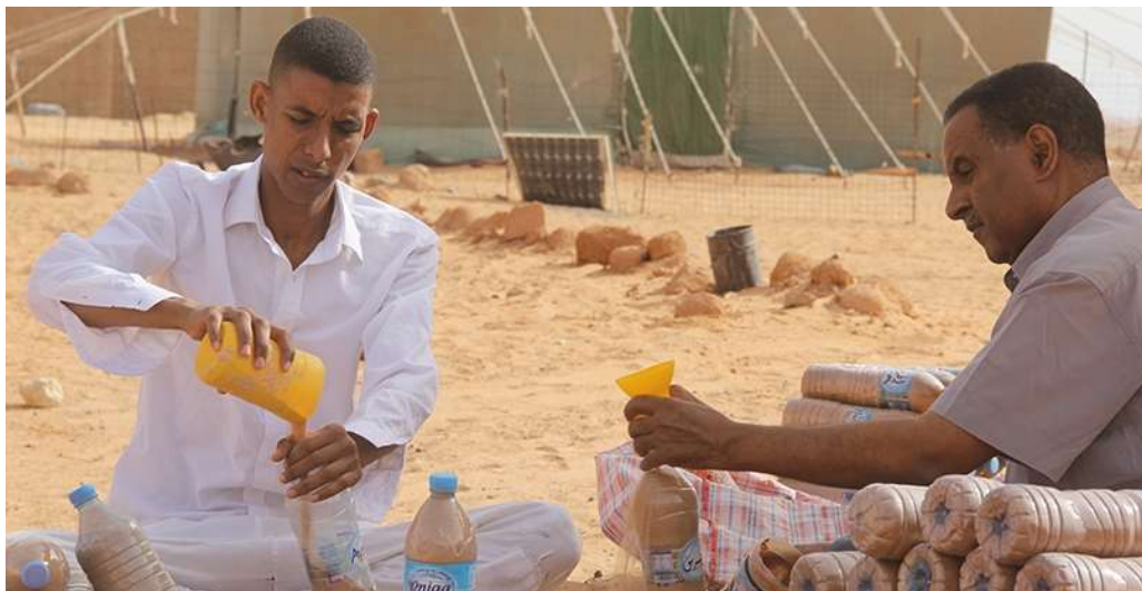
Figure 4.4-1. Filling the collected bottle bags with sand, converting the bottles to a construction material, (World-habitat, 2018).
