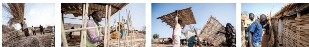
Figure 4.3-12. Bamboo Thatching and grass roofing for existing shelter upgrade, in South Sudan, (Global Shelter Cluster, 2019)
