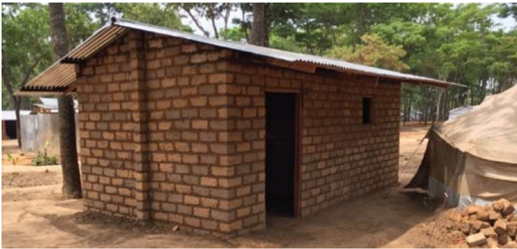
Figure 4.3-22. Air dried Lime stabilized adobe Transitional shelter next to the Tent shelter that the family was living in, Nduta refugee camp, (Shelterprojects, 2017)
