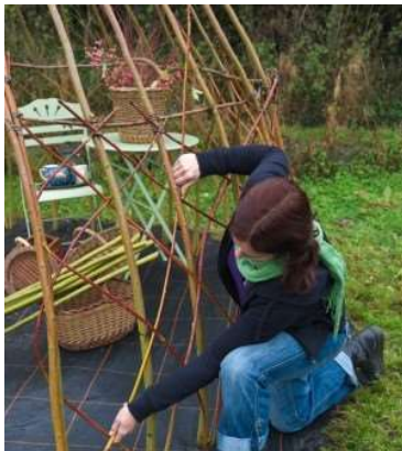
Figure 5.9-14. Woven living willow weeds for living structure. (Stocken, 2021).
