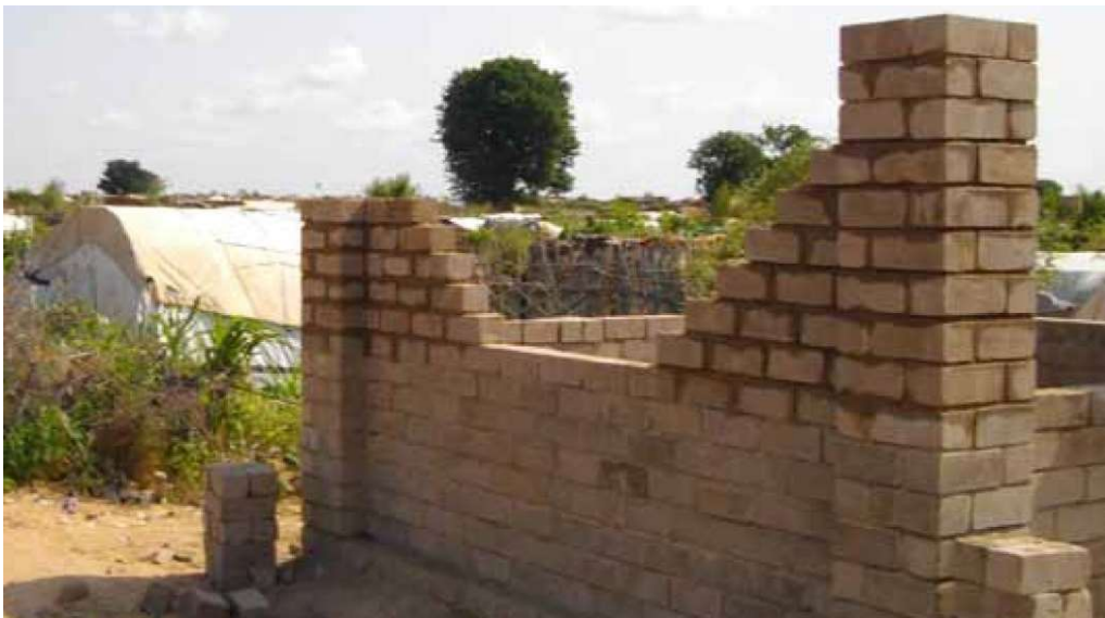
Figure 4.3-25. Upgrading settlements from tents to houses using (SSBs). (UN-Habitat, 2012)
