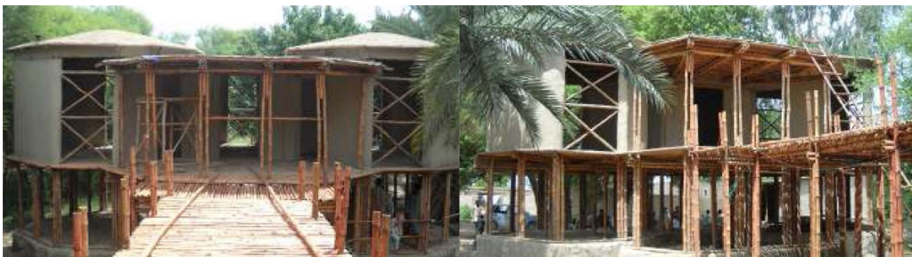
Figure 4.3-36. Raised on stilts bamboo structure combined with mud, Health center and primary school, Village Darya Khan Sheikh, (Shaikh and Uthero., 2011)
