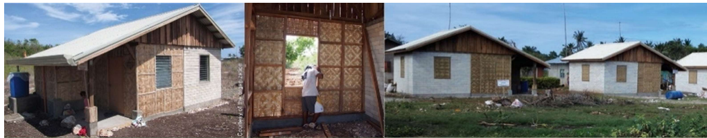
Figure 4.3-47. the hybrid core houses with lightweight extension, Philippen, 2015 to 2017 (Global Shelter Cluster, 2019).
