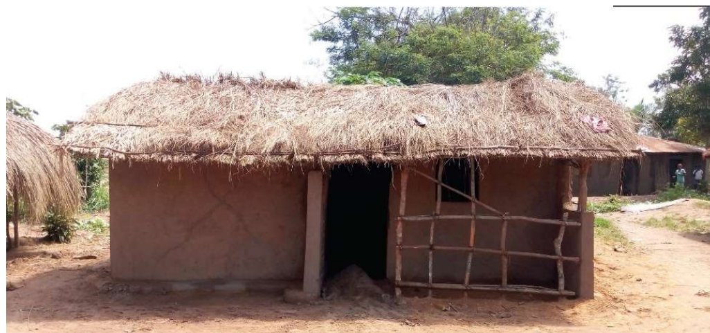
Figure 4.3-13. Cost effective shelter built with locally available materials, Congo 2018, (Global Shelter Cluster, 2019)
