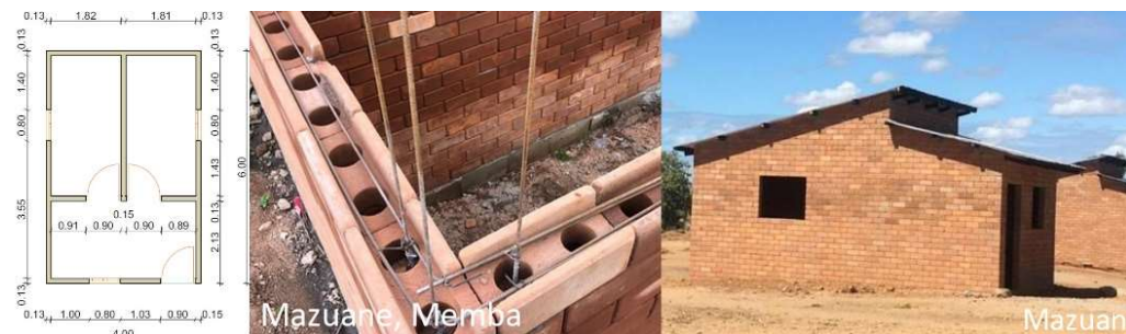
Figure 4.3-44. CSEB interlocking blocks Permanent shelter in Mazuane, Memba (Shelter Cluster, 2021).
