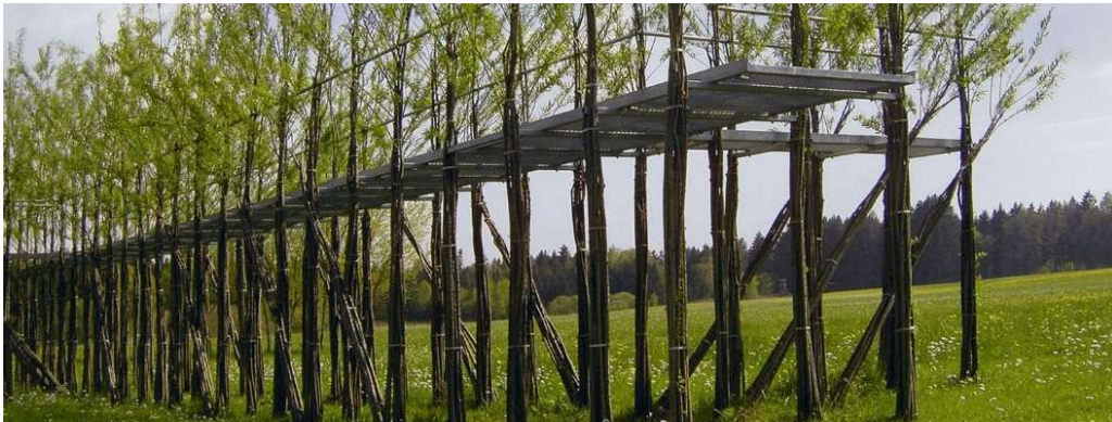
Figure 5.9-17. The experiemental structure of baubotanik foot bridge by (Ludwig and Schonle, 2005)
