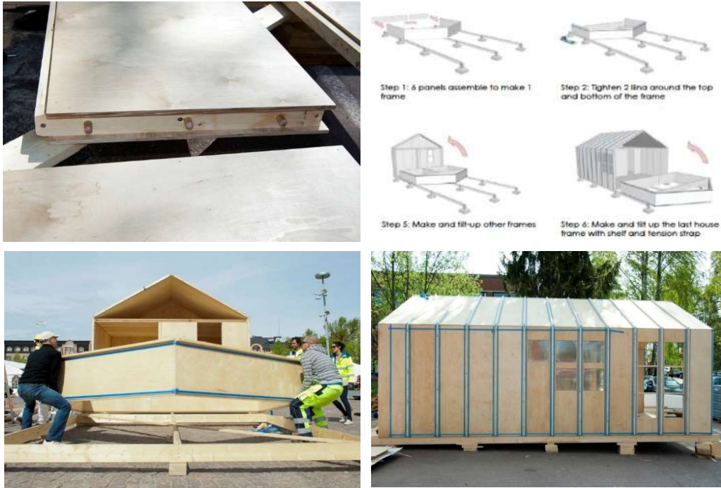
Figure 5.9-4. The assembly process of the prefabricated panels and the stacked frames. (Meinhold, 2011).
