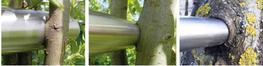
Figure 5.9-18. Development of steel handrail connection with living trees over 5 years, (Future Architecture, 2016).
