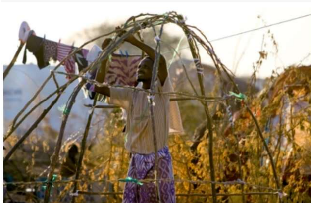
Figure 5.9-15. framed woody structure for emergency shelter, in Dadaab, Kenya, 2008 (UNHCR, 2019a).
