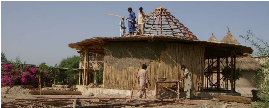
Figure 4.3-10. Plastering the Thatch walls with mud, By Architect Yasmeen Lari, (Andreea, 2020)
