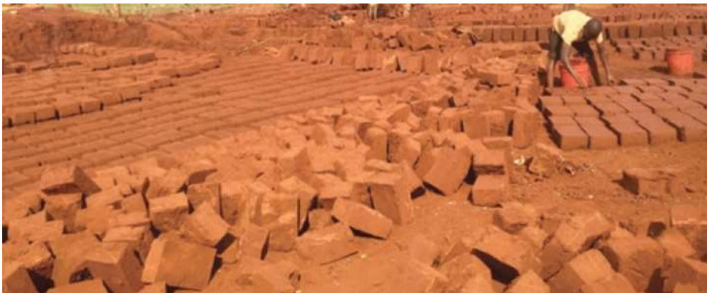
Figure 4.3-23. Air dried adobe, Lime stabilized, in Nyaragusu refugee camp, Tanzania, (Shelterprojects, 2017)
