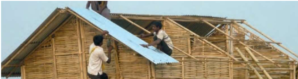
Figure 4.2-6. CGI roofing for transitional bamboo shelter in Nepal, (IFRC, 2016)
