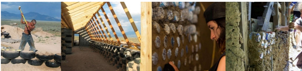
Figure 4.4-4. The building process using (earth, old tyres, and used Glass and cans. (Reynolds, 2021).
