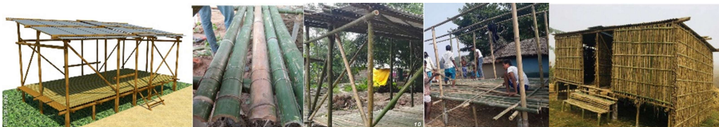
Figure 4.3-5. Bamboo framed shelter, with bamboo mats for walls, Nepal floods, 2017, reference (Global Shelter Cluster, 2019).
