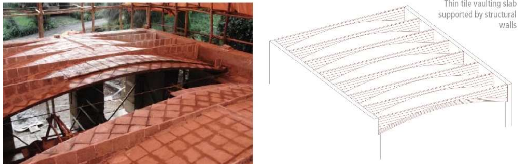
Figure 4.3-29. Single curved low rise thin tile vaulting slab supported by load bearing walls, (Ball et al. , 2014)
