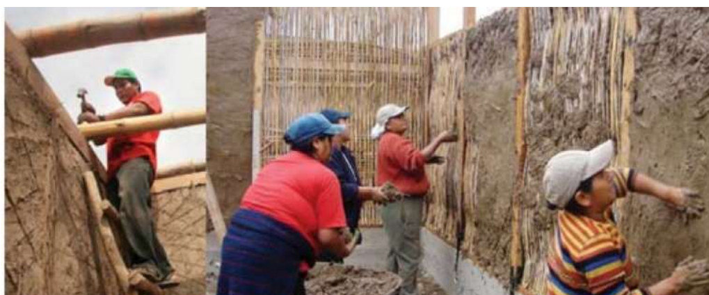
Figure 4.3-11. Plastering woven thatch wall, Quincha mejorada, Peru, (Shelter Center, 2012)
