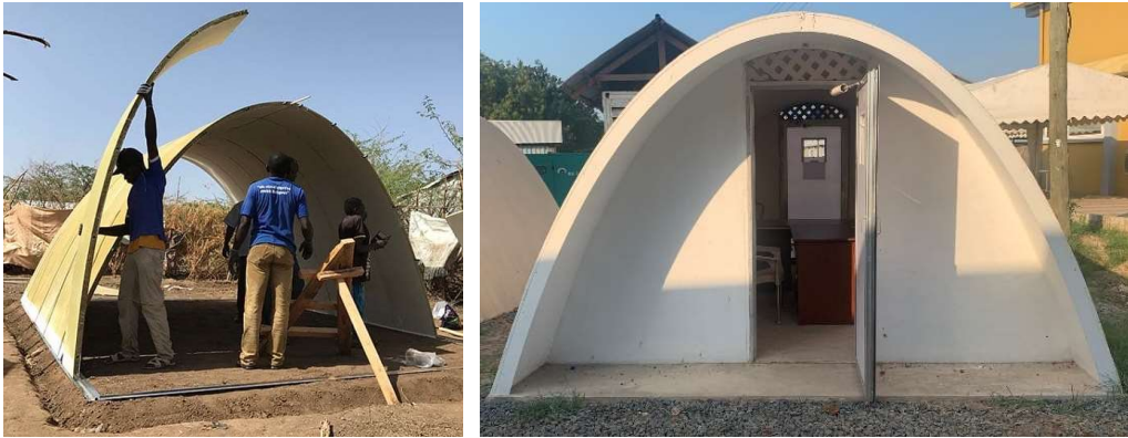
Figure 4.5-1. Bending rock wool light weight panels, performing Humanitarian shelter, (Life-shelter, 2013).
