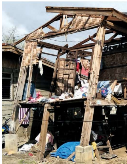
Figure 4.3-3. Example of racking effect after Tayfoon Haima, 2016, Philippines, by (IFRC, 2016).
