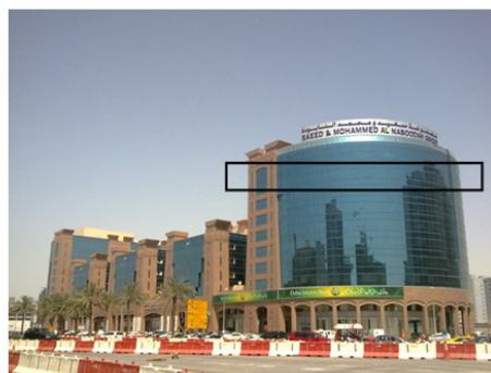
Figure 1 Photo of office building used for the simulation (Author)
